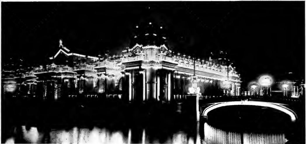
FIG. 21.—A NIGHT EFFECT NEAR ELECTRICITY BUILDING.
